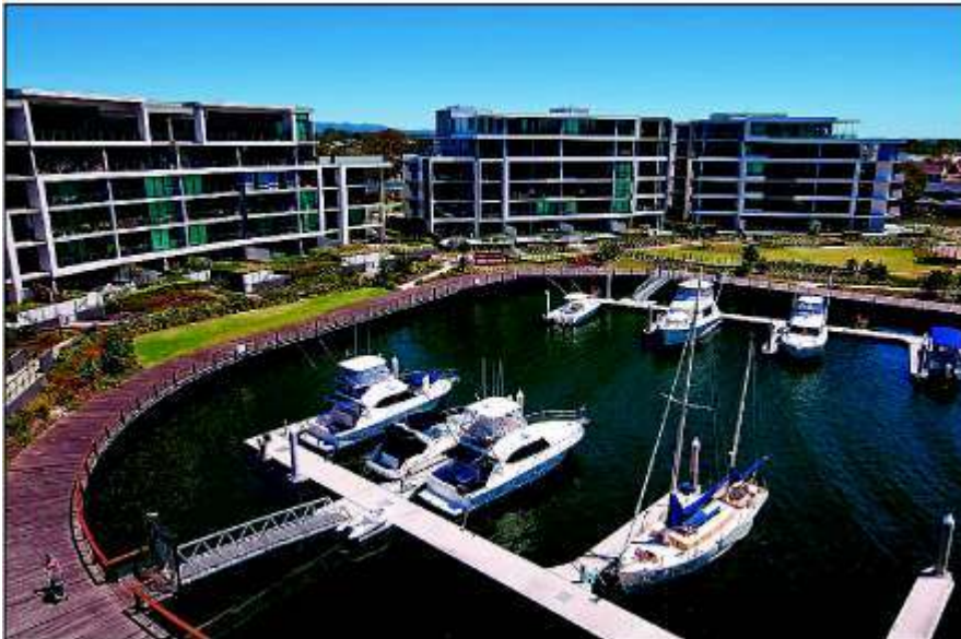
The Marina precinct at Stockland's Allisee development in Hollywell
