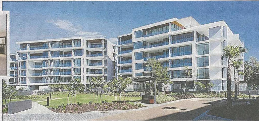
Construction of the Maricel (left) and Bijou buildings completes Allisee at Hollywell
